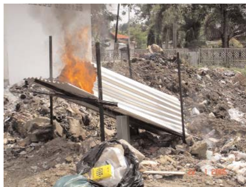
Photo 4: Incline Plane Incinerator constructed by EH Team
