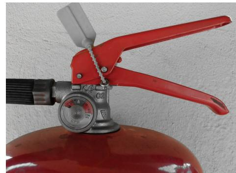
If a fire extinguisher does not have a pressure gauge, it may have to be weighed to ensure it is still full.
