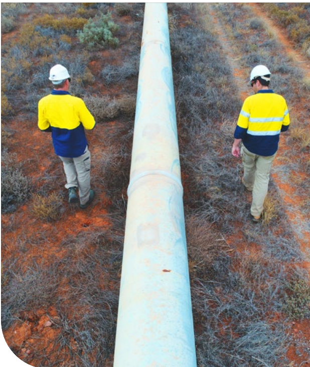
Pipeline inspection in outback Australia
