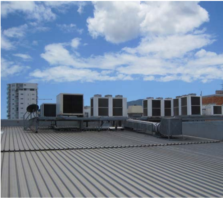
Example of noise-emitting equipment on a roof near residential units in the CBD
